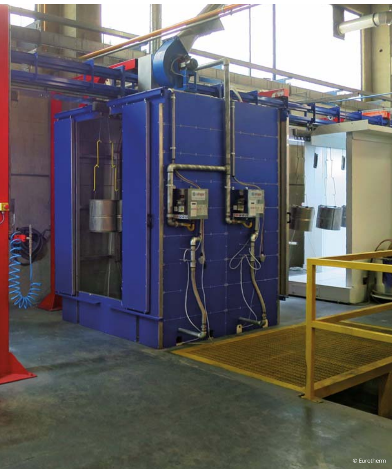
From right to left: Booth for application of primer, IR oven for gelation and application of top coat.
